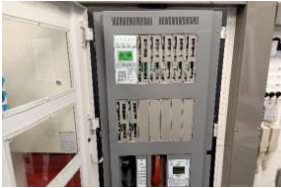
Fire Alarm Control Panel
